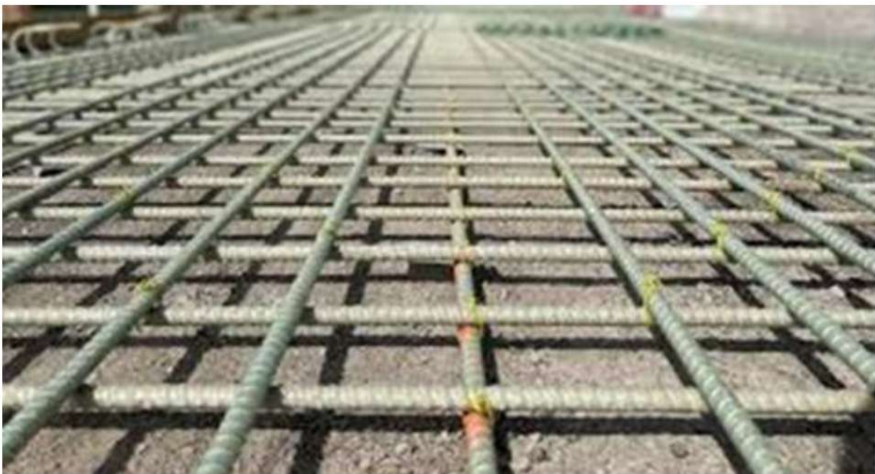
Use of FRP bars enhancing durability and reducing lifecycle emissions in infrastructure projects.
