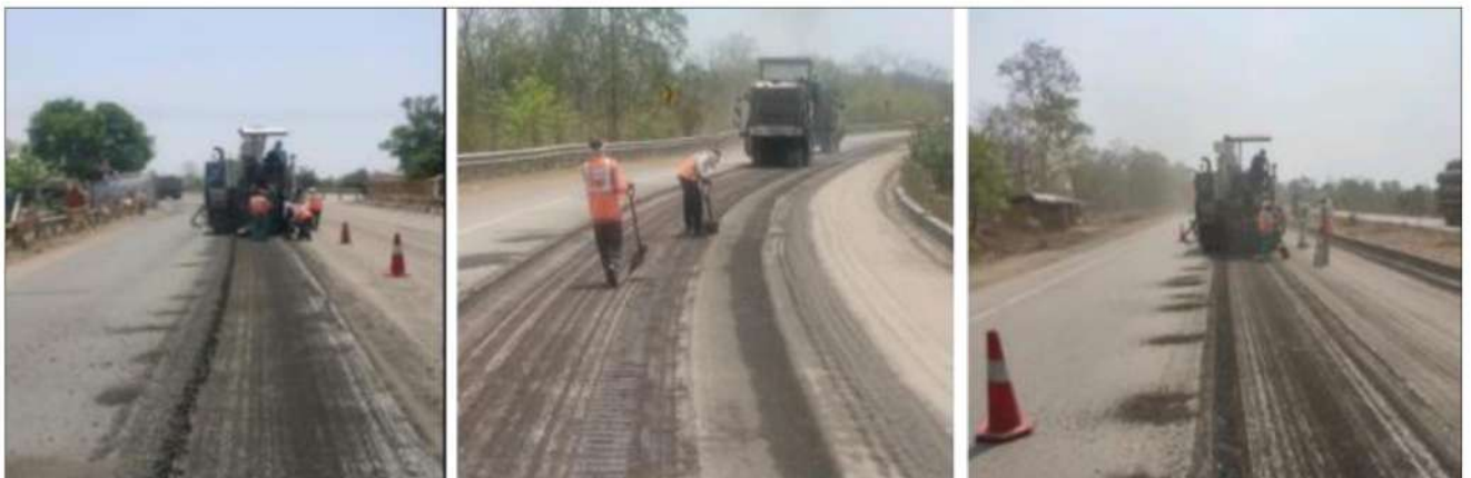
Images: Recycled milling material at project sites.
