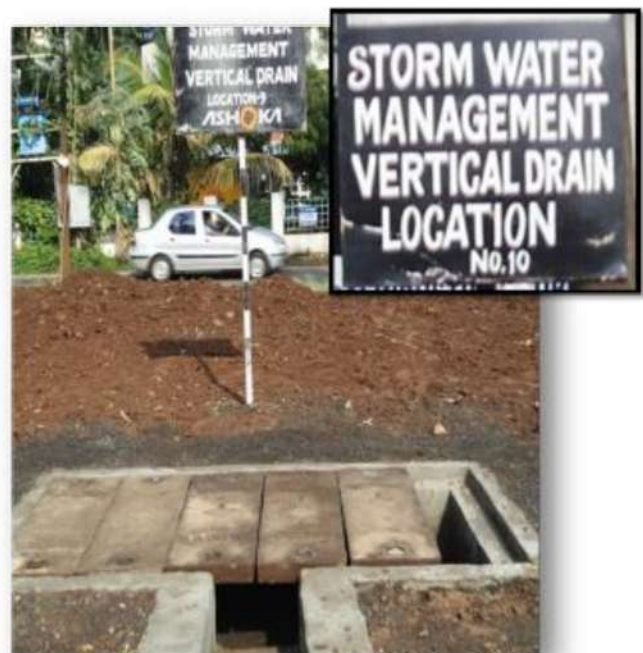
Rain Water Harvesting: Recharge Pit
