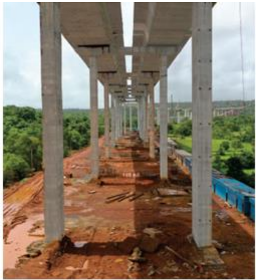
The elevated corridor consists of numerous piers that reach height of up to 40 meters.
