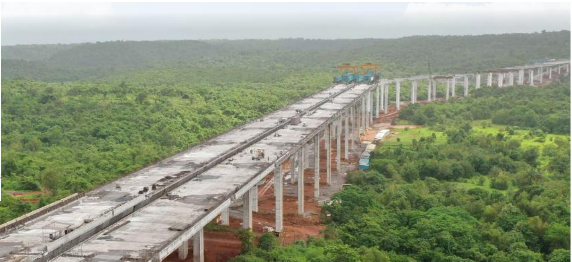
The elevated corridor consists of numerous piers that reach height of up to 40 meters.
