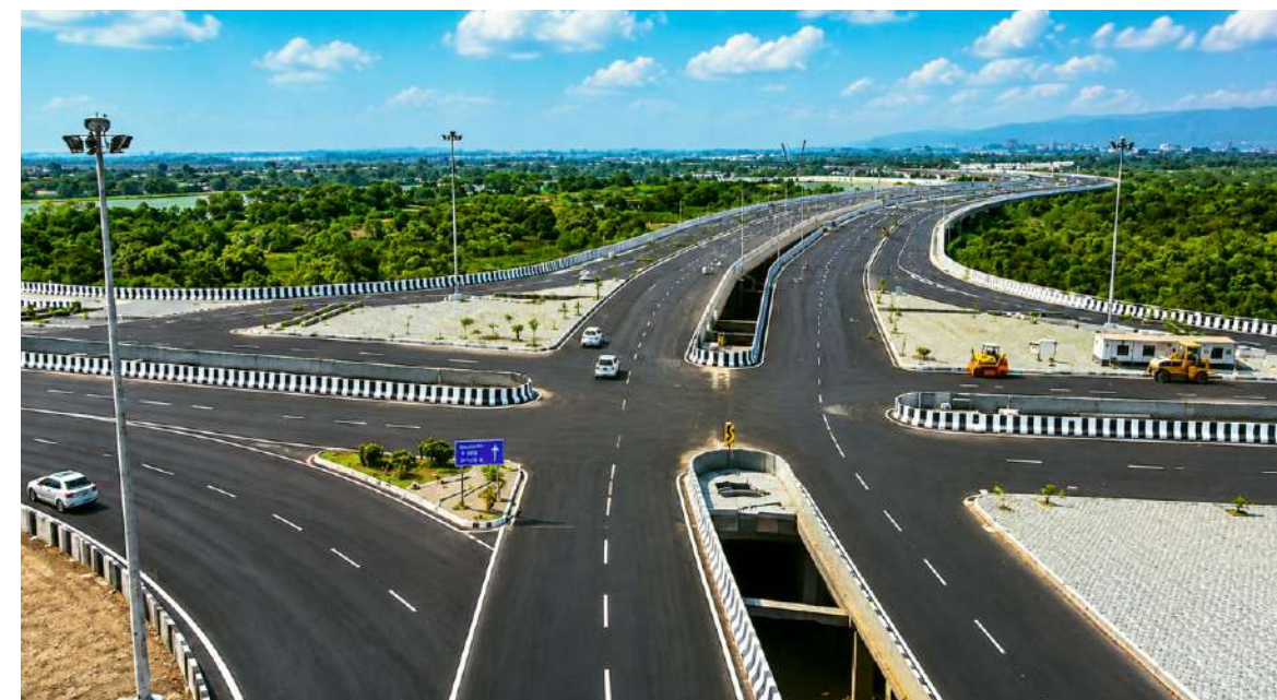
Stilt Bridge SBR-9, Eastern Connectivity - Maharashtra
