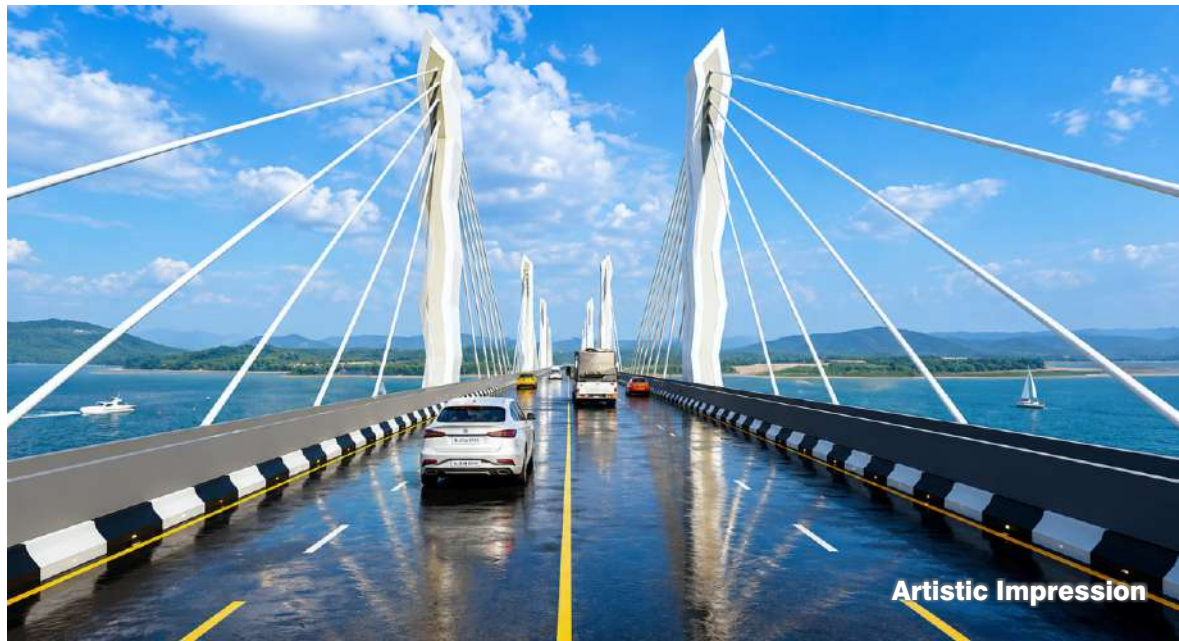
Jaigad Cable-Stayed Bridge - Maharashtra Crossing Jaigad Creek with a 40-metre navigational clearance, improving connectivity to Ganapatipule Beach
