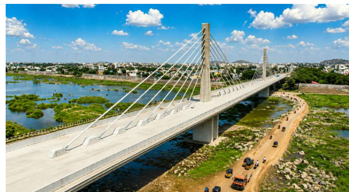
Khammam Cable-Stayed Bridge - Telangana
