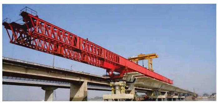
The team began working on the Second bridge simultaneously and completed it in 364 days. The pictures depict various stages in the construction of this bridge which has been built using 360 concrete segments and stands on 21 piers comprising of 178 pile foundations.
