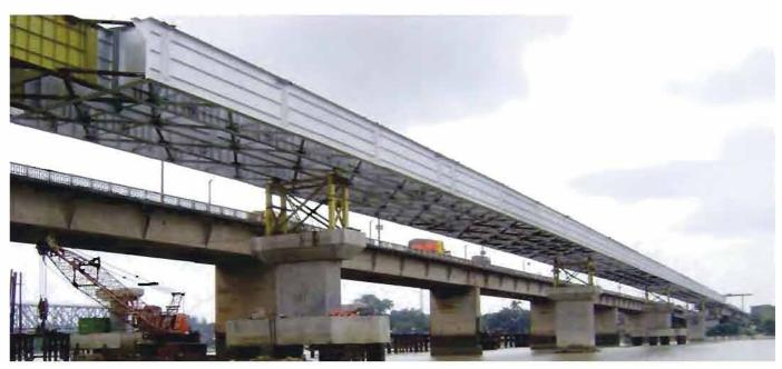
Ashoka Buildcon Limited completed the First bridge in 305 days. The pictures show the launch of the massive steel girder assembly weighing over 1700 MT and 323 metres in length. The nature of the river bed, water flow conditions and the wind force were some of the major difficulties that endangered the success of the project.
