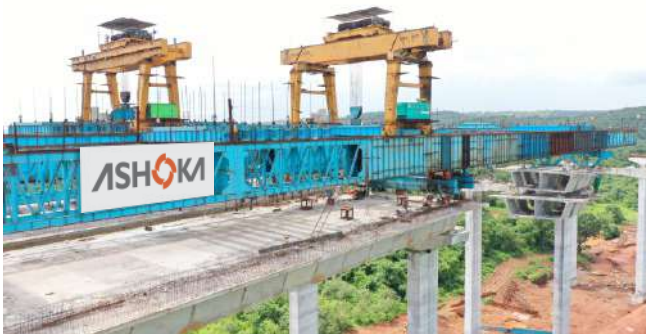
Mopa Airport Link Road
